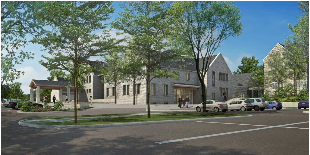
Atrium entrance to the new Formation Building with porte-cochere to the left.
